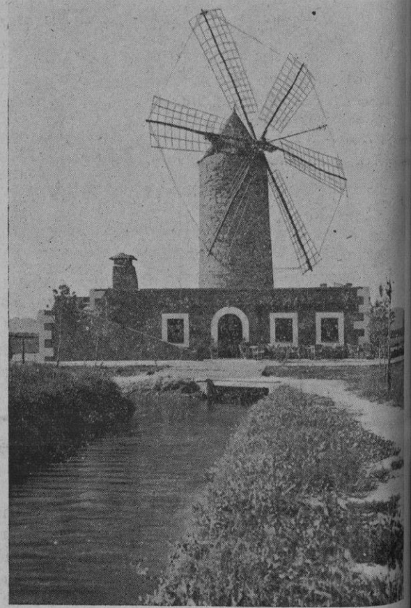
The club house of the only golf course in Mallorca
