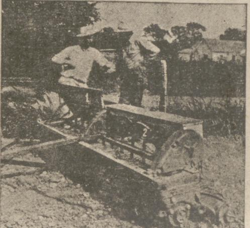
Mechanical sowing machine with hopper. The hopper, with the lid raised (1), regulates the seed rate (2) and the rollers (3) of the three rows. In page 8 an article by agronomist Roque de Laburu.
