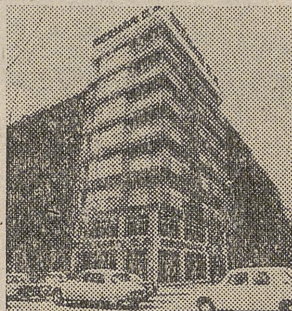
EDIFICIO RESMAN (VIA LAYETANA, 185) (ESQUINA A DIAGONAL)
