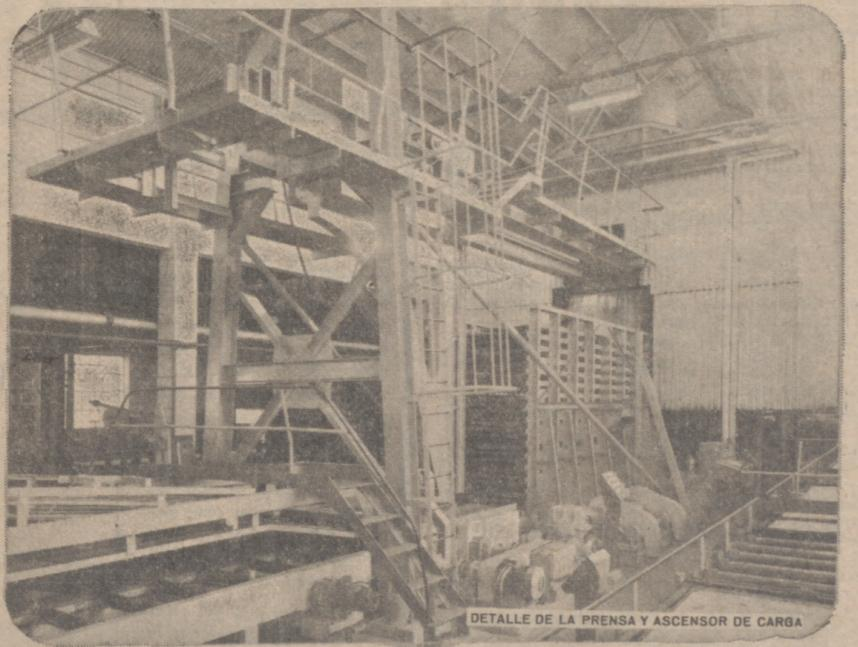
DETALLE DE LA PRENSA Y ASCENSOR DE CARGA
