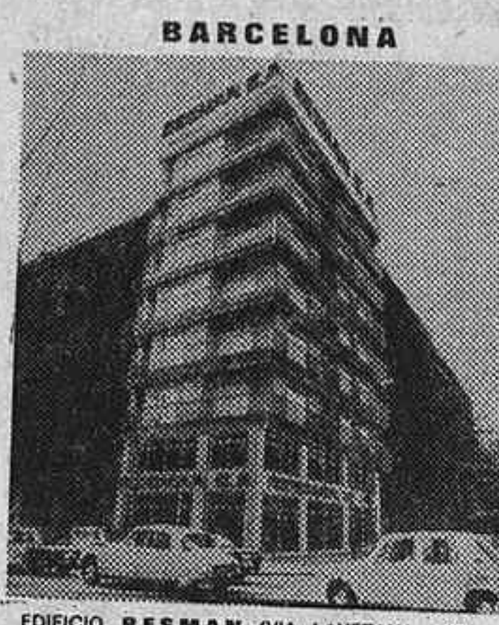
EDIFICIO RESMAN (VIA LAYETANA, 185) (ESQUINA A DIAGONAL)
